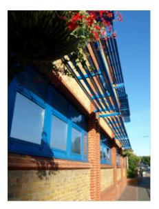
Figure 8. Brise soleil, Tonbridge Police Station (Photograph courtesy of Kingfisher Louvre Systems: <u>http://www.kingfisherlouvres.com/brise\_soleil.html</u>)
